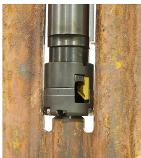
Remove membrane from between tubes
