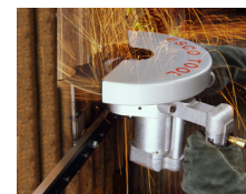
The boiler tube panel saw works on the same track as the straight-thru models.
