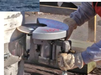
Scoring concrete pilings for height trimming. Concrete Cut-Off Blades are available in Diameters of up to 14".
